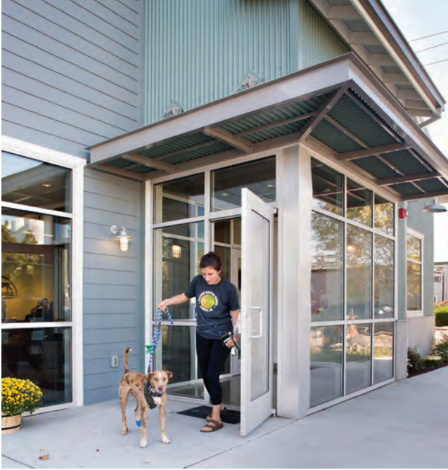
A vestibule—two sets of doors—can prevent a loose pet from escaping but also, if set up correctly, allows the front desk to control who can enter. This vestibule is at Adobe Animal Hospital of Petaluma, California.
